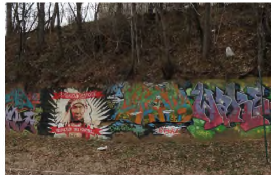
E. Retaining wall
