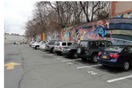
F. Retaining wall
