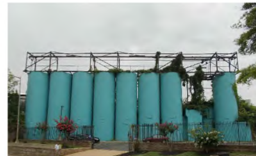
J. Silos on Rhode Island Ave.
