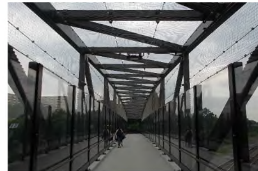
F. Metro Bridge
