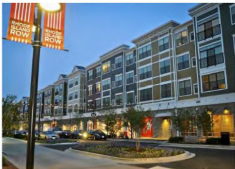
D. Rhode Island Avenue Row Apartments
